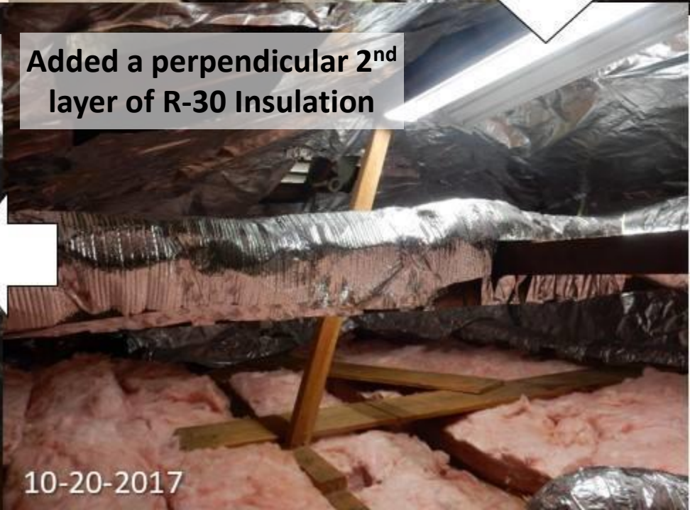
Finished with a layer of Radiant Barrier
