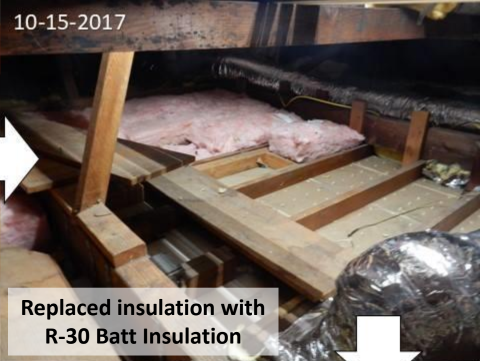
Added a perpendicular 2 nd layer of R-30 Insulation
