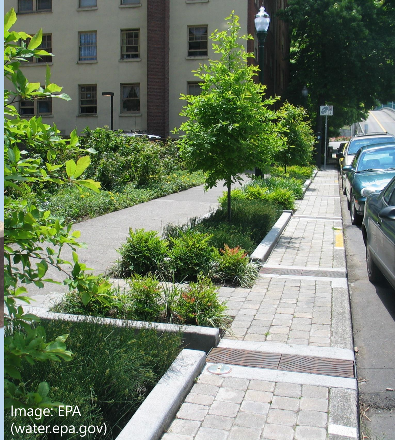
Fig. 2.1 3D View of Stormwater Planter Philadelphia Green Streets Design Manual
