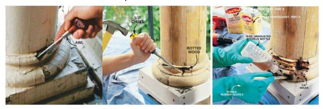
**3.** Mix the two parts of consolidant according to the manufacturer's directions. Then squeeze the consolidant into the 1/4-in. holes and onto the wood in the repair area. Work it into the wood with a small disposable brush. Continue this process until the wood is saturated.
